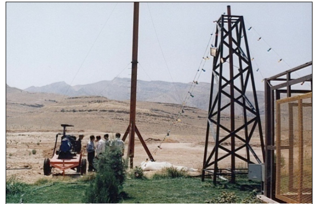
Figure 3.9: Electricity Generation from Shiraz Landfill Gas (pilot project)
