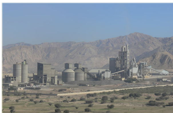
Dashtestan Cement Plant, Bushehr Province
