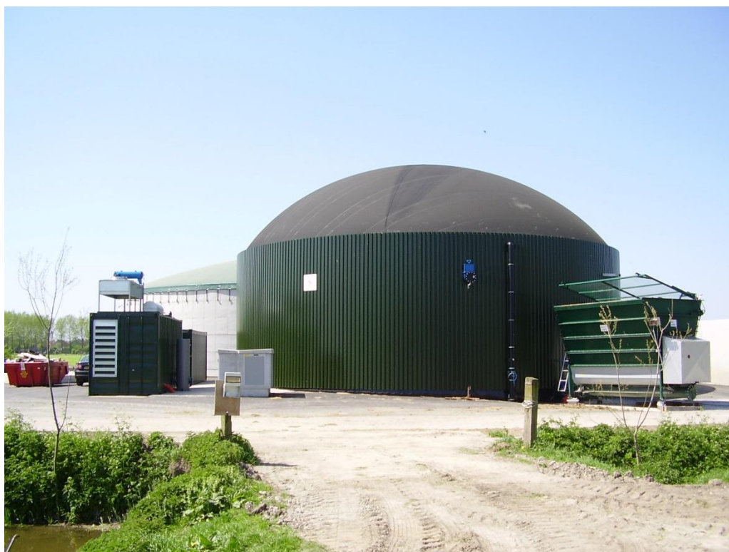
Figure 6: Digester with EPDM rubber cover (adopted from www.biogasnieuws.blogspot.nl/2011_08_01_archive ).
