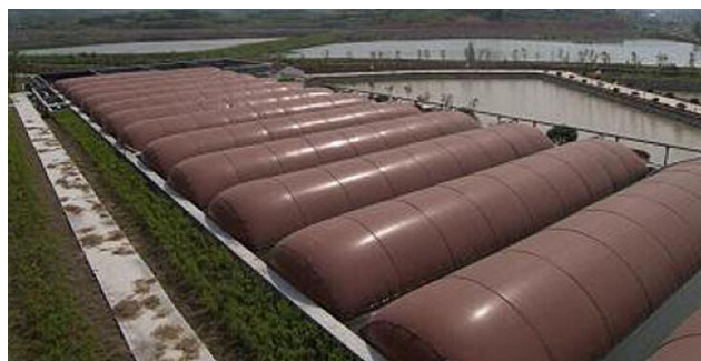
Figure 13: Gas bag with single membrane (adopted from www.alongenvirotech.en.made-in-china.com ).
