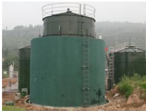
Figure 11: Floating gas holder (adopted from www.alibaba.com ).
