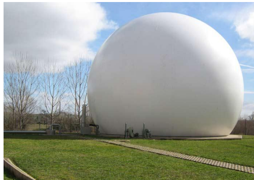
Figure 12: Gas bag (inner and outer membrane) (adopted from www.gticovers.com ).
