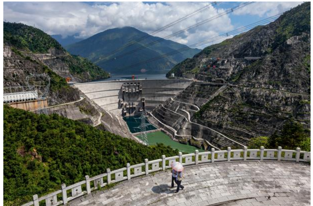
Xiaowan Dam, Mekong River, China
