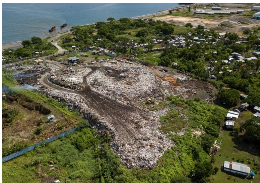
Figure 53. Aerial view of Honiara's landfill
