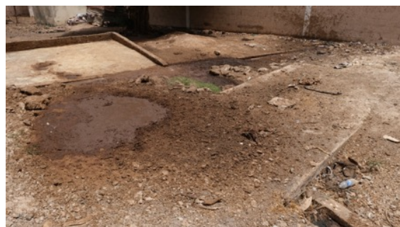
Slaughterhouse's exploded wastewater system
