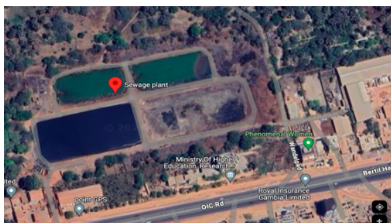
Sewage plant near ECOSOIL
