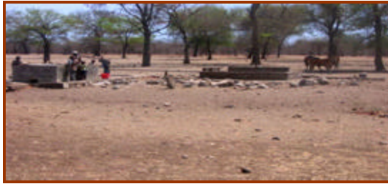
Only a few boreholes are functional. Most are broken down due to lack of capacity for maintenance
