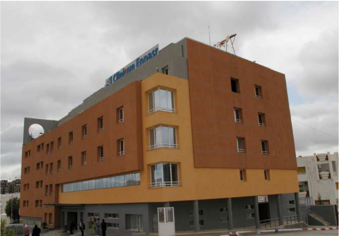
Tertiary Sector Office Buildings, Ennasr Private Clinic © Eric Thauvin / ADF
