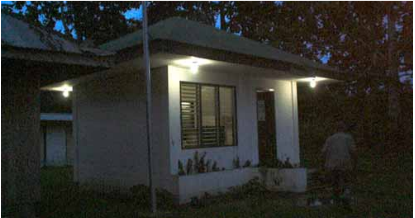
Lighting homes through solar home systems. Project: Accelerating Community Electricity Services using Solar (ACCESS) – the Philippines.
