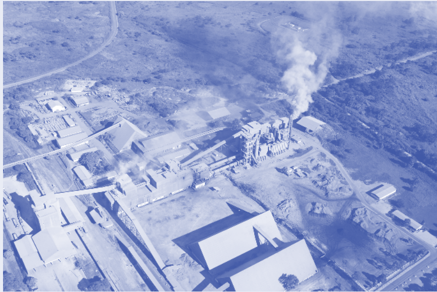
Copper ore treatment plant, Ndola/Copperbelt, Zambia. © Cordier Sylvain/BIOSphoto/Still Pictures.
