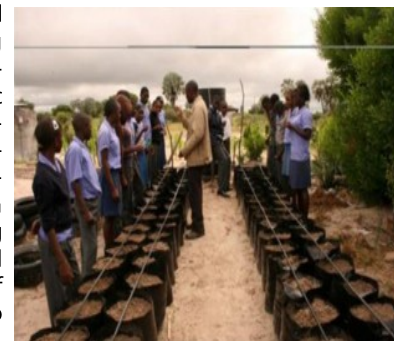
Setting up a micro drip irrigation system at the Onamulunga Combined School. Vegetable seed is planted in 40 litres poly bags allowing the user to control a local soil/ compost/manure mixture in the bags and thus controlling soil fertility and soil quality. Photo: Andreas Tweendeni/CES for UNDP CBA
