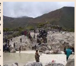
Workers clearing the main channel from the Thorthormi Lake to reduce water levels
