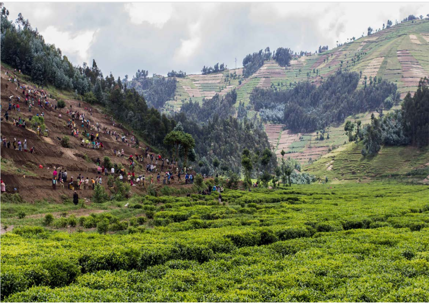
Photo: Local community members participating in the construction of graded terraces to control for soil erosion in Rwanda. Supported by LDCF. Credit: Rik Moors/One UN Rwanda
