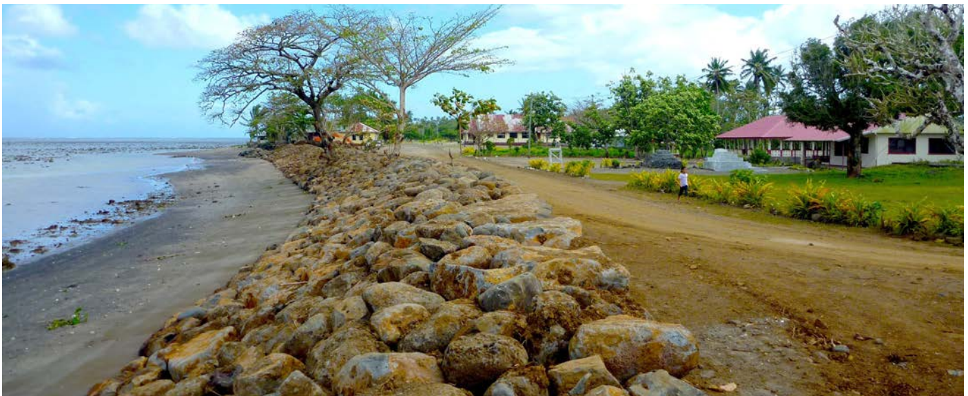
Photo: Sea walls constructed for coastal protection in Samoa. Supported by LDCF. Credit: UNDP Samoa
